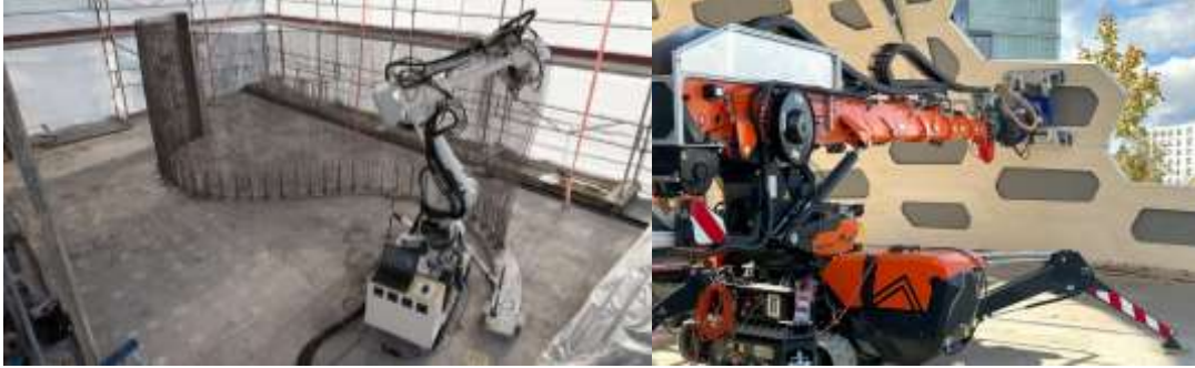
Figure 2:. Application examples of mobile large payload robots in construction: a) wheel-based industrial robot for mesh bending and welding on site [7] ; and b) mobile robot in application to assemble timber wall and roof surface components for the Buga pavilion [8].
