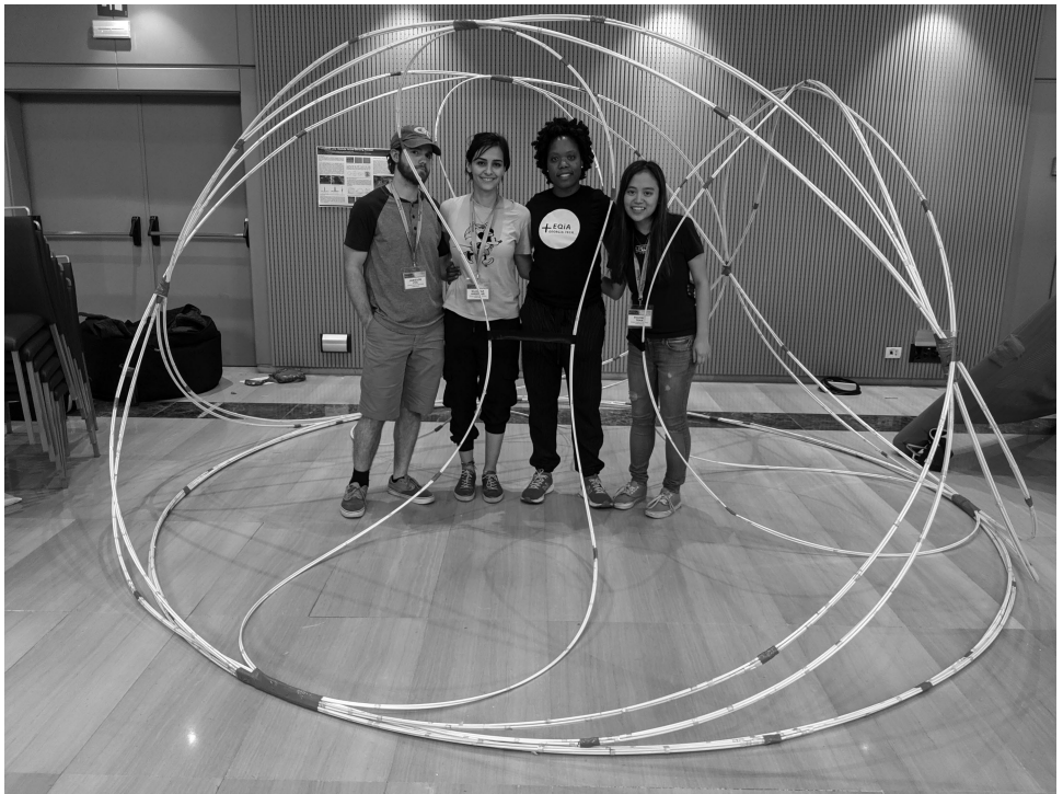
Figure 17.2 The Infinite Line Active-bending pavilion – designed based on material behavior and fabricated using techniques from wire-bending on exhibition at International association for shell and spatial structures (IASS) in Barcelona, Spain (2019).
